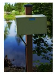
The post mount cabinet must be attached to a sturdy post or to a vertical wall with electrical service. If possible, install rubber between the post and the cabinet to reduce vibrations.
