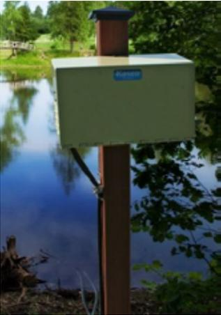
The post mount cabinet must be attached to a sturdy post or to a vertical wall with electrical service. If possible, install rubber between the post and the cabinet to reduce vibrations.
